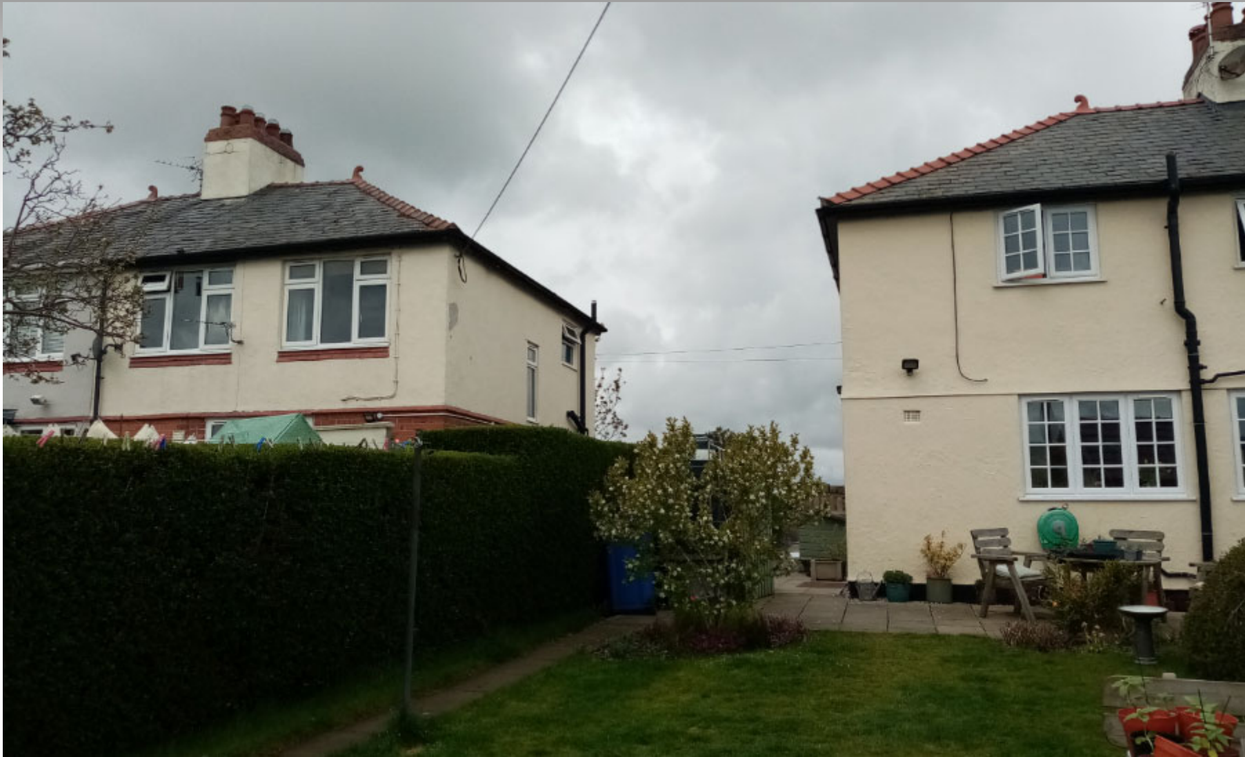
Rear of property and other neighbouring property
